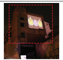
D: WALL SURFACE D2: TOP OF RAMP PAVED AREA
