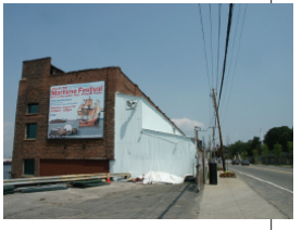
C: OPEN ASPHALT PAVED DOCK AREA
