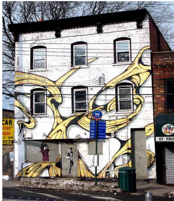
Re-visioning a Boarded Up Building at 57 Victory Blvd
