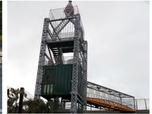
Ferry Terminal Viaduct
