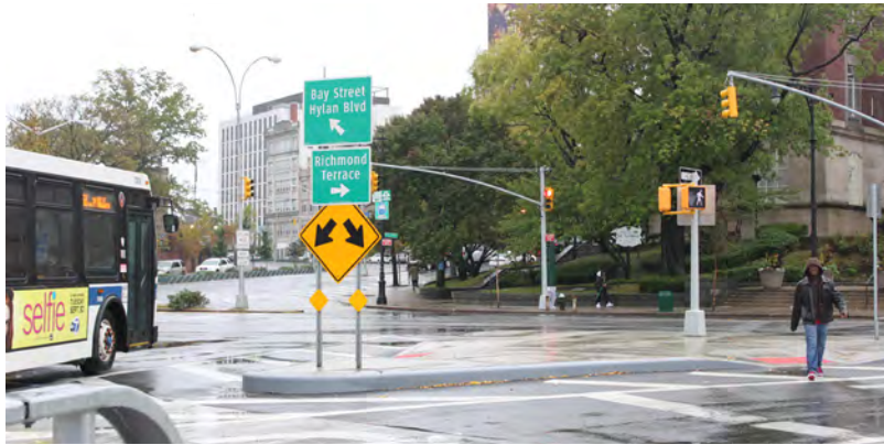
Bay St. & Richmond Terrace Intersection - St. George
